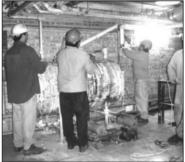
Boiler Demolition Crew
