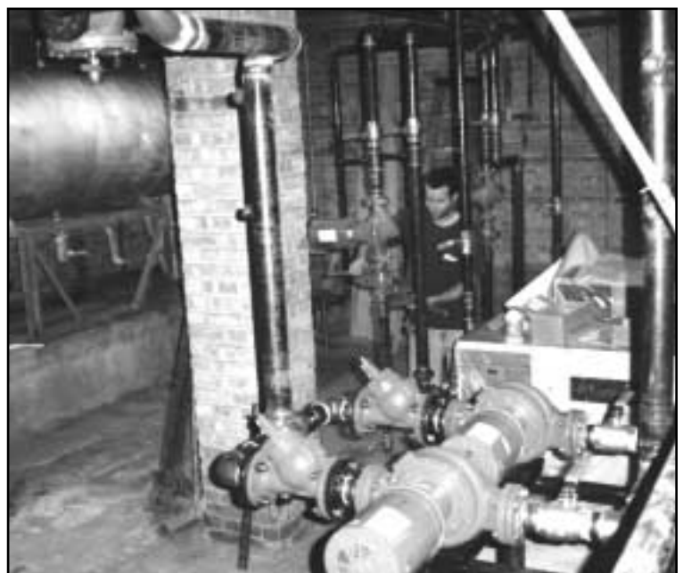
Installation of New Boilers
